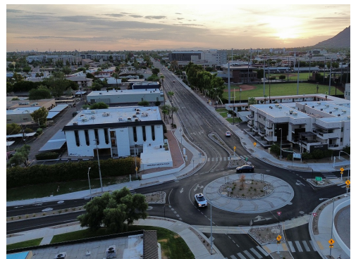
Miller Road and Osborn Road roundabout.
