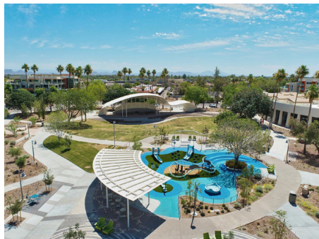
Civic Center (Lake|Flato and Dig Studio).
