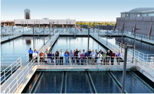
Graduates of Scottsdale Water's Citizens Academy at Advanced Water Treatment Plant
