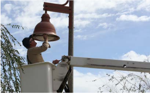
Facilities Staff install lights in Downtown Scottsdale
