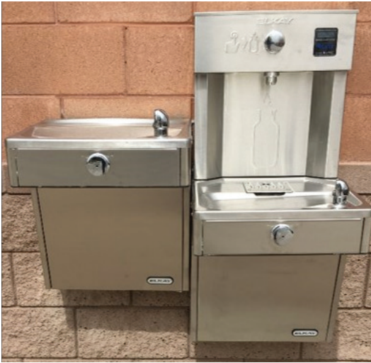
Newly installed drinking fountain replacement
