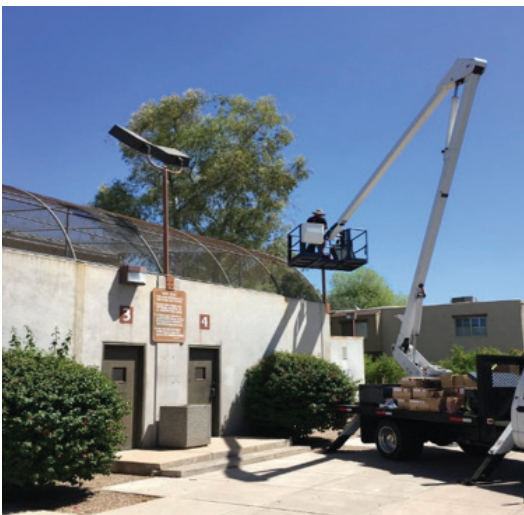
Facilities crew replaces lighting with more LED fixtures
