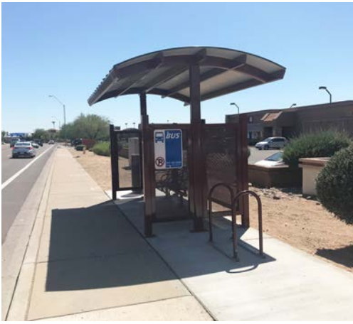
Bus shelter at Pima and Via de Ventura
